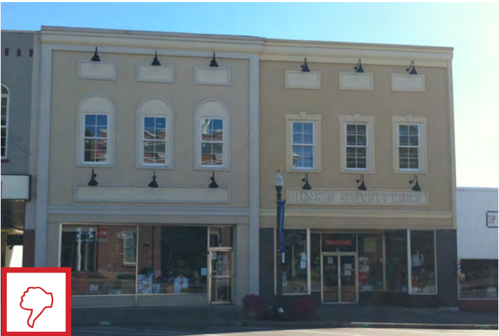
These historic buildings have been inappropriately resurfaced and detailed with E.I.F.S (Exterior Insulation Finishing System); E.I.F.S and stucco are inappropriate building materials for Downtown Winchester
