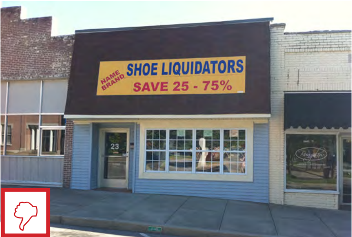
This asphalt shingled mansard type roof is inappropriate for Downtown Winchester commercial buildings; note inappropriate use of vinyl siding, residential vinyl windows and inappropriate signage
