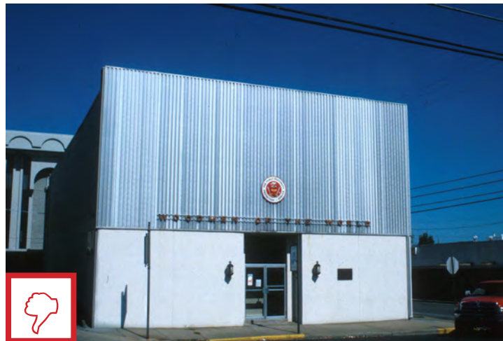
This civic building lacks appropriate facade detailing and windows and is clad inappropriately with industrial metal siding and E.I.F.S.
