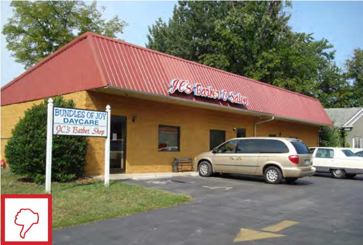
This metal, overhanging false mansard roof is inappropriate for downtown Winchester; note also the inappropriate use of painted concrete block as a facade material
